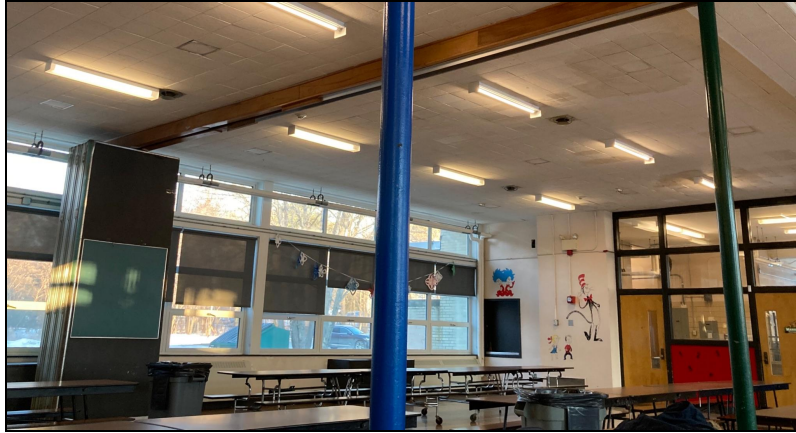
Figure 3: Chandler Magnet’s ground floor cafeteria room (2/15/2022)
